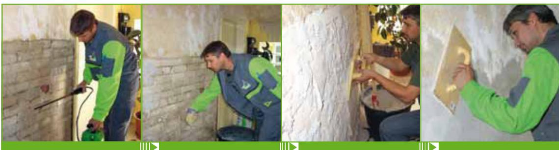
**Remove old plaster. Fill breakouts and holes with KÖSTER Repair Mortar. Spray KÖSTER Polysil® TG 500 onto the surface to block salts and harden the substrate.**
